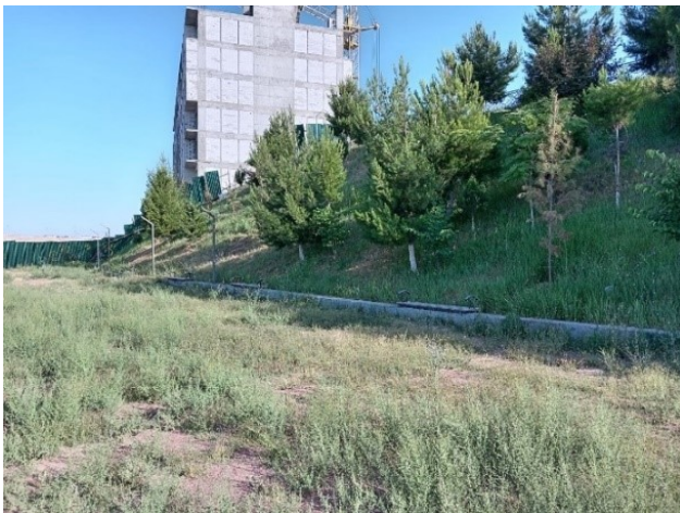
Figure 4. View of multi-storey residential buildings under construction from G'irvonsoy Street.
