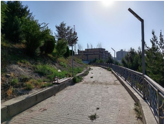
Figure 3. View of multi-storey residential buildings under construction from I. Karimov Street.
