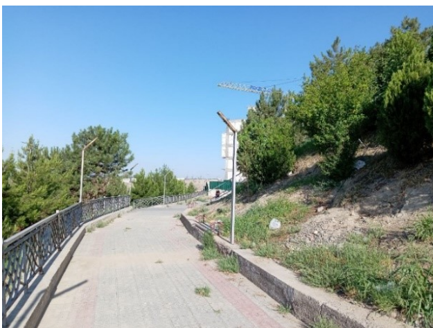
Figure 5. Existing condition of the site
